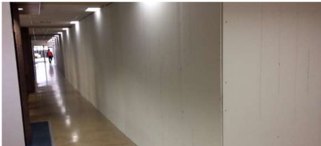
Figure 3 Temporary Enclosure to Protect Corridor from Construction Area.
