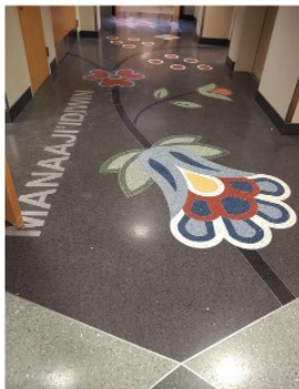
Figure 3 Terrazzo - adjacent HEAPR project
