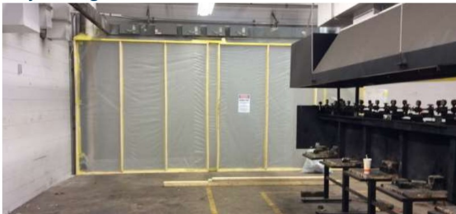
Figure 2 Abatement Enclosure at Former Welding Area.
